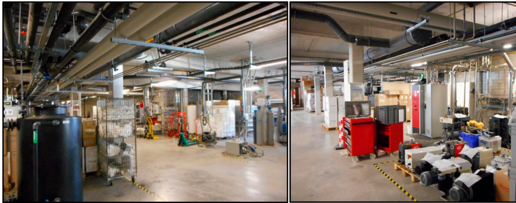
Figure 1. Industrial environments considered in this paper. The walls, metallic pipes and machines generate undesirable clutter that challenge the long-range detection and wireless reading of zero-power sensors for the monitoring of pressure.
